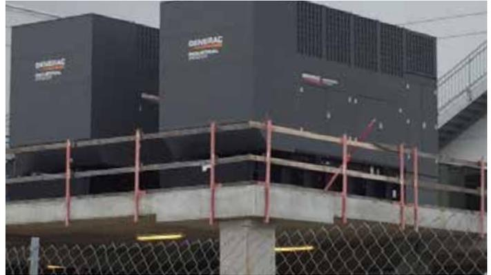
As a result, a raised platform design is typically used with new facilities, not retrofits, due to the complexity and costs involved with moving utility components to ensure electrical distribution to the generators.
