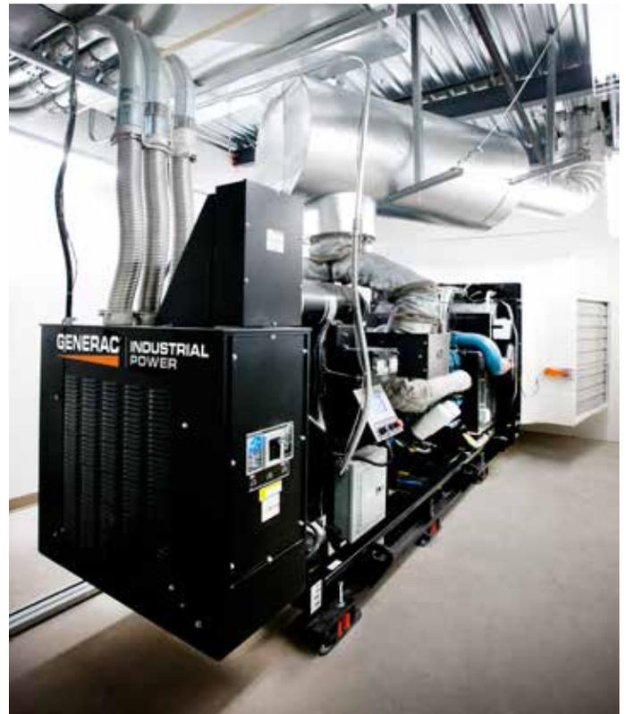
be removed from the area to prevent overheating. High heat taxes the engine which may trigger a shutdown sequence to prevent damage to the engine and generator. Ventilation is typically done through the use of an air inlet, air outlet/exhaust fan, and/or other ventilation openings. The air inlet must be capable of moving
