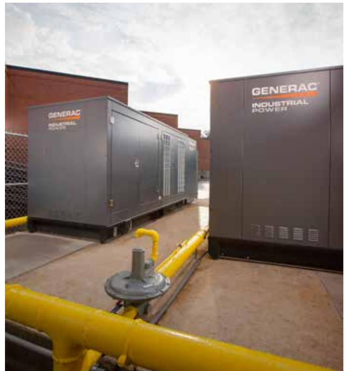
At the same time, optimal placement of the generator(s) is equally important with outdoor applications as it is with indoor applications. Facility managers or customers may prefer the generators to be located in an area that is "behind the scenes" to maintain the design aesthetics of the structure. This may not be the best option based on site-specific conditions such as wind and weather patterns, accessibility and code compliance.
