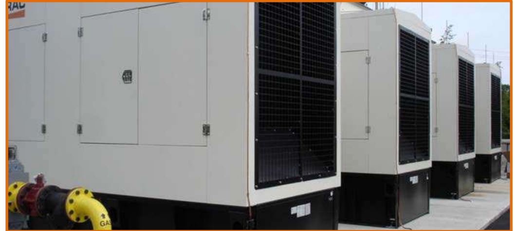
134 Air Force Guard Base – 4x600kW Bi-Fuel – Alcoa, TN
