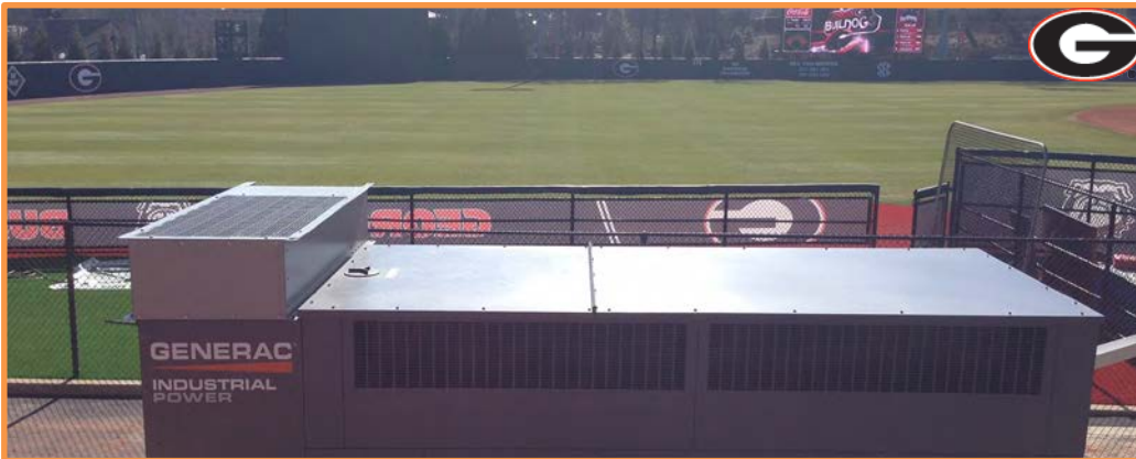
UGA Foley Field –Diesel Genset w/integrated Load Bank – Athens, GA
