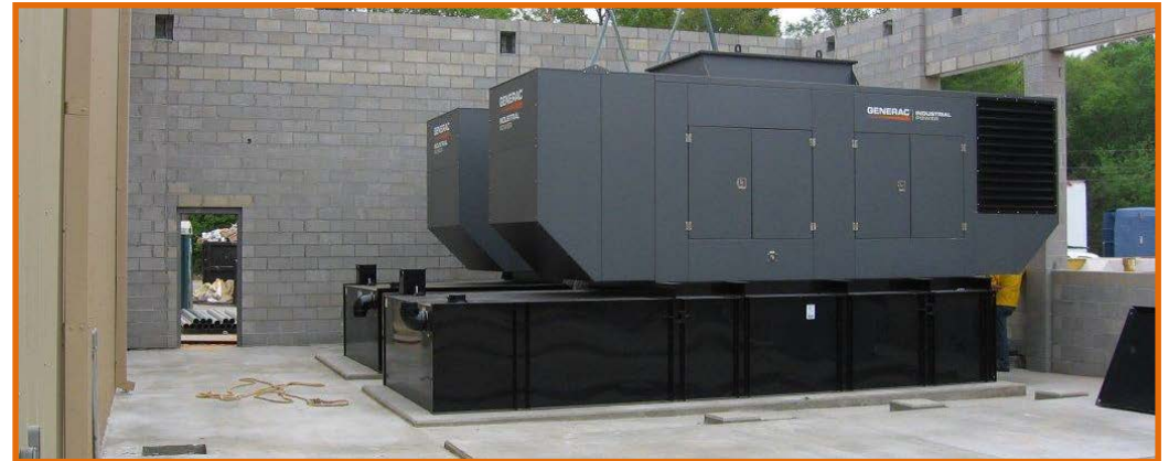
T-Mobile Switching Station – 2x600kW Bi-fuel with space to grow – Mobile, AL
