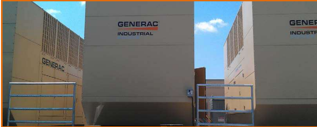
T-Mobile Switching Center – 3 x 1,000kW Gemini – Nashville, TN
