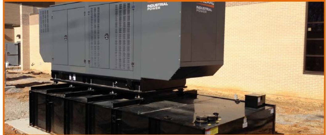
Healthsouth Acute Rehab – 400kW w/ 1900G Tank & Seismic – Chattanooga, TN
