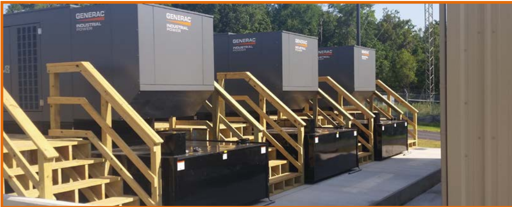
Bay County WTP – 3x500kW Diesel, Step-up 4160V Transformer – PCB, FL
