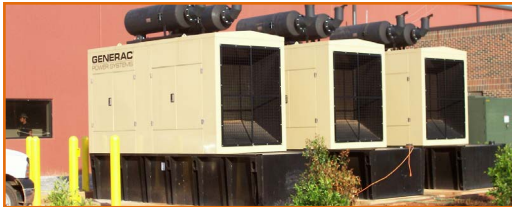
CR Bard – 3 x 600kW, Soft Loading SE ATS – Madison, GA
