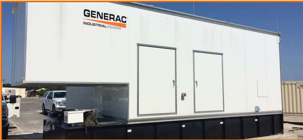
NAS – 750kW Diesel w/custom enclosure – Jacksonville, FL
