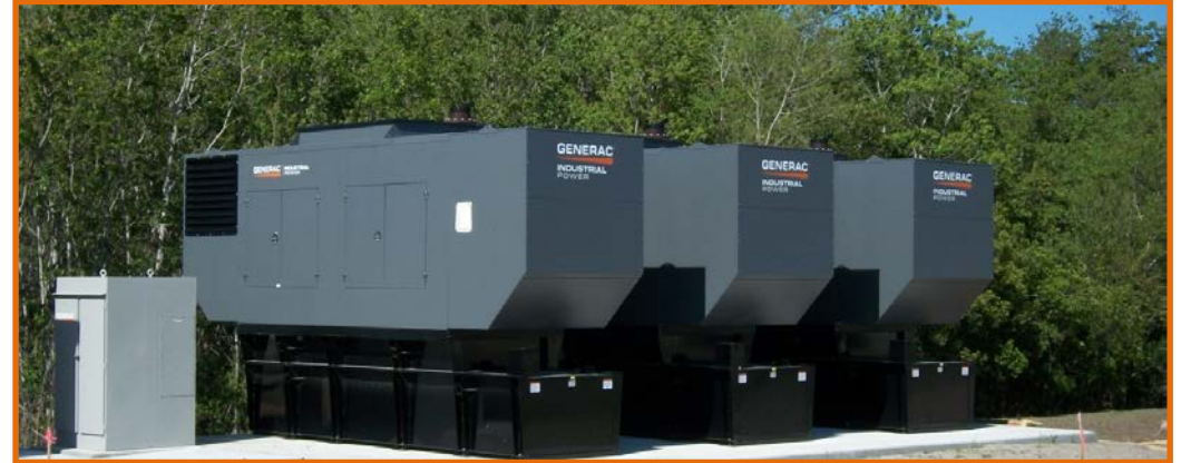
3x500kW Water Treat., 150kW Lift Station, 150kW Main Bldg – Panama City, FL
