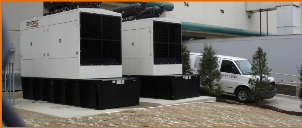
Cardinal Health DC – 2 x 500kW with 1600A ATS – Memphis, TN
