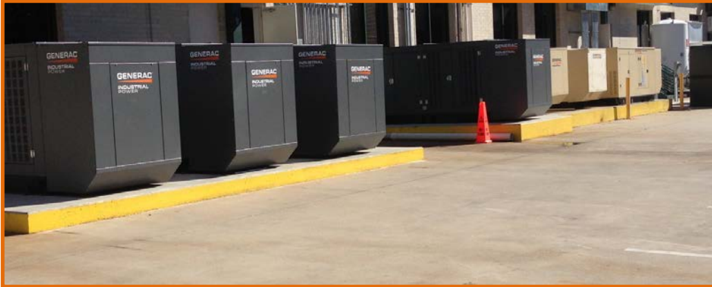
Arris Bank/Data Center – 4x200kW expanded with 4x300kW – Norcross, GA
