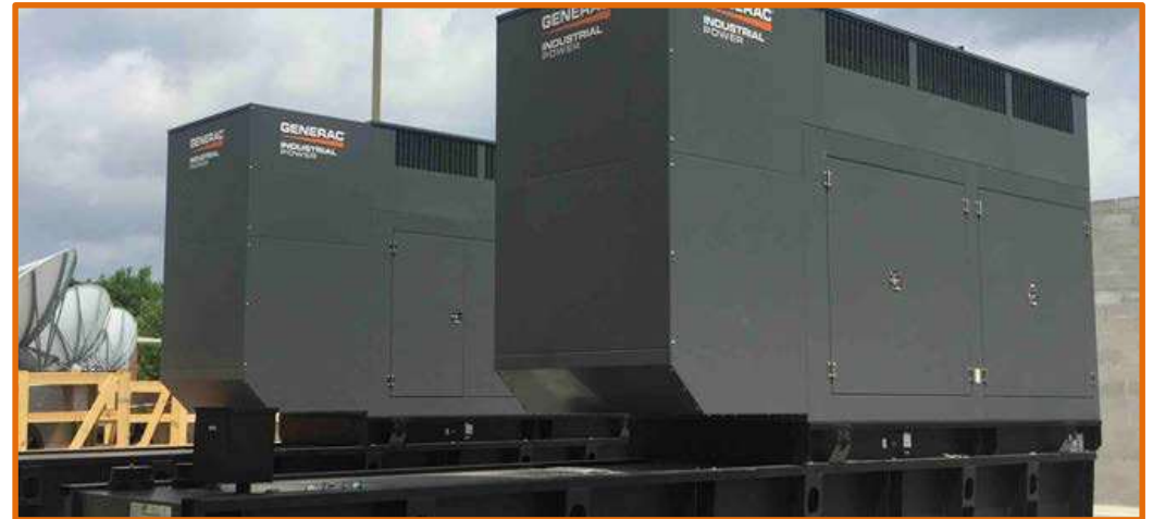
Comcast Cable – 2x400kW Diesel – Huntsville, AL
