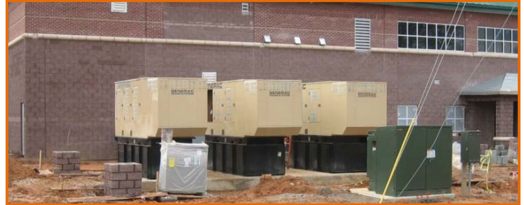
Forsyth County 911 & Sheriff – 4 x 400kW Diesel – Cumming, GA
