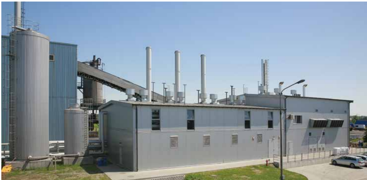
Condensation plant - Sokołowie Podlaskim - Poland.
